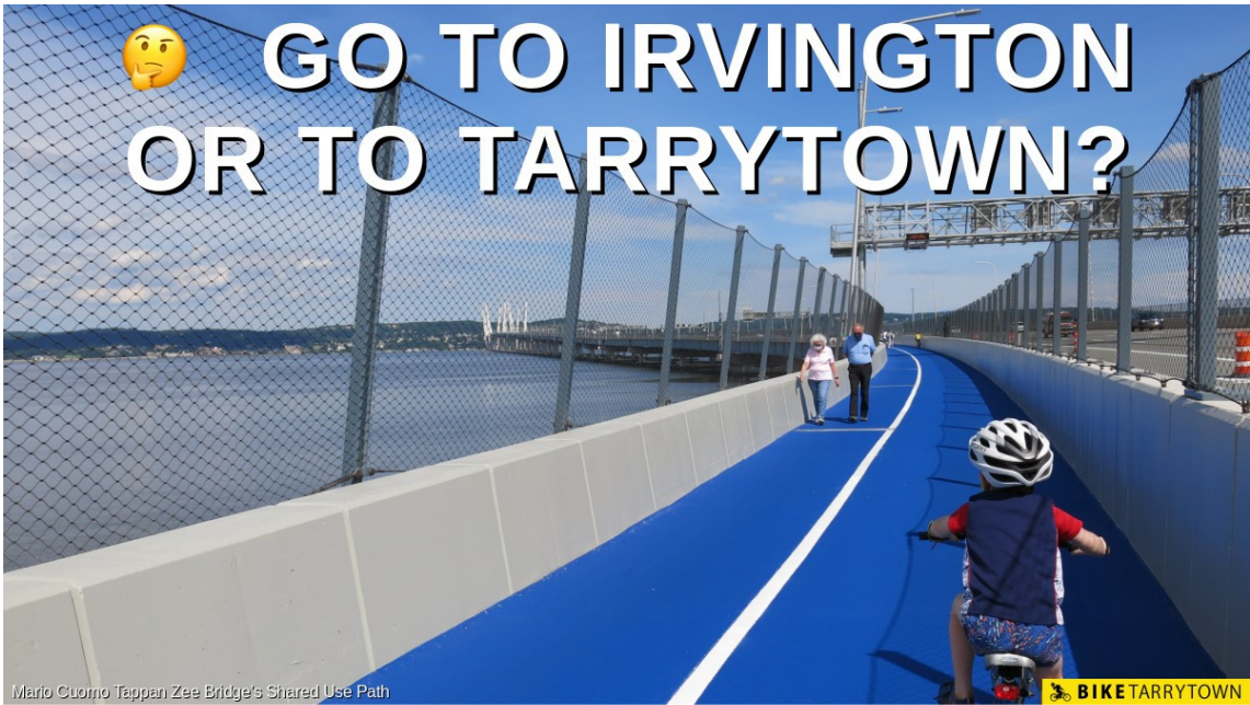
Mario Cuomo Tappan Zee Bridge's Shared Use Path
