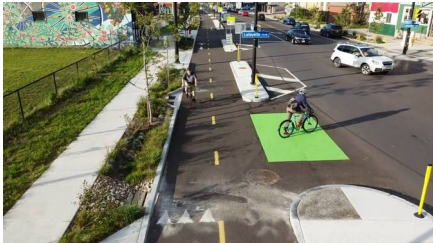
Route 266 (Niagara St), Buffalo DOT Region 5. Completed November 2021. Note: design integrates many driveways. Credit: GObike Buffalo
