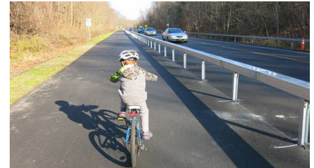
Route 100, Briarcliff Manor DOT Region 8. Completed November 2020. Note: box beam median barrier; strong protection, only needs a little width. Credit: Bike Tarrytown
