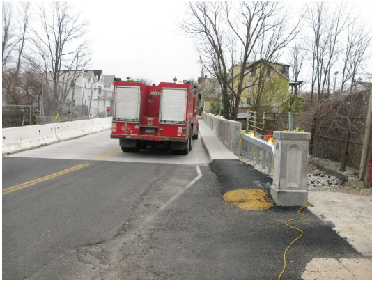
Vehicles can easily swipe people walking. b) "Ramp" doesn't meet ADA requirements.
