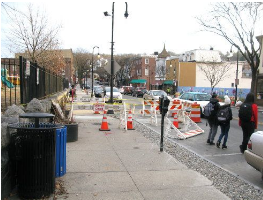
example of sidewalks closed for construction without a safe bypass. ( More examples. )
