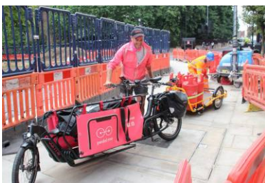
Road work materials being hauled by a cargo bike. (@pedalmeapp)
