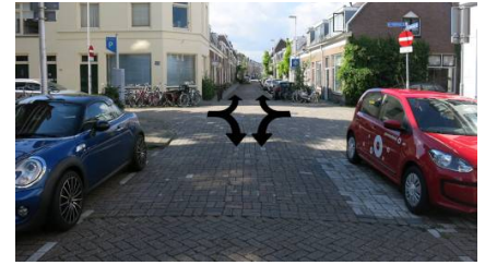
Alternating one ways allow local travel while eliminating motor vehicle through traffic.
