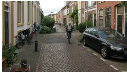
Perfection: narrow street, chicane (created by parking shifting sides), speed hump, bollards, pavers.
