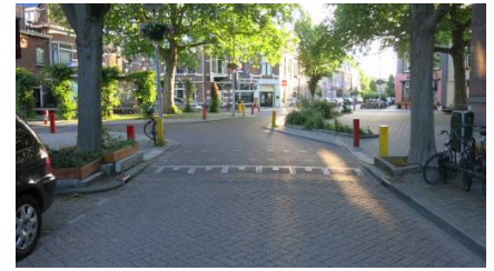
Curbs extensions, bollards and trees make people drive more carefully through this intersection of multiple two-way streets. A lovely place to relax with three cafes.
