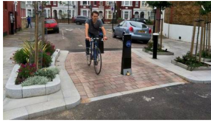
Greenery and bollards encouraging human scale mobility by keeping through traffic out. (@HaringeyCyclist)
